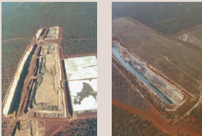
Bottle Creek mine site before and after rehabilitation
